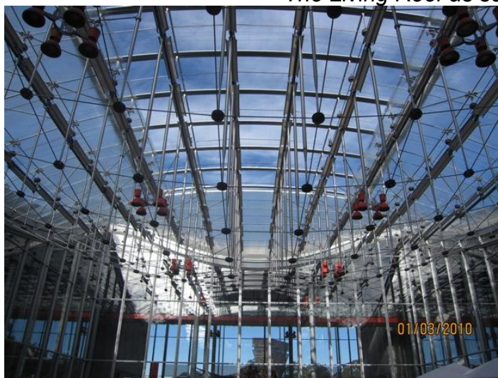
Left: Roof of the Cafeteria
