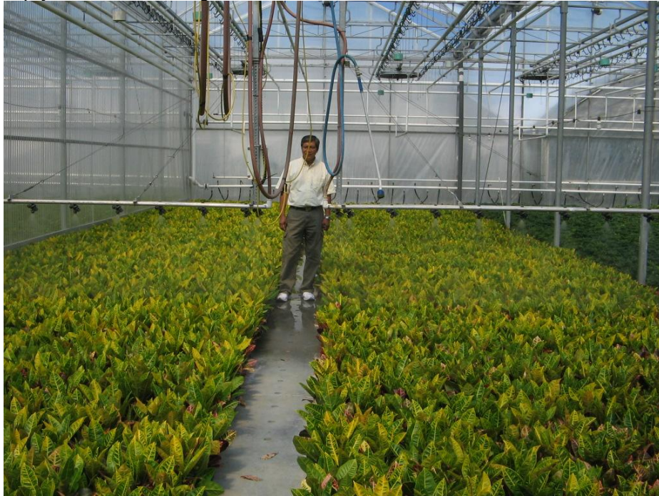
Irrigation boom at Rainbow Greenhouses
